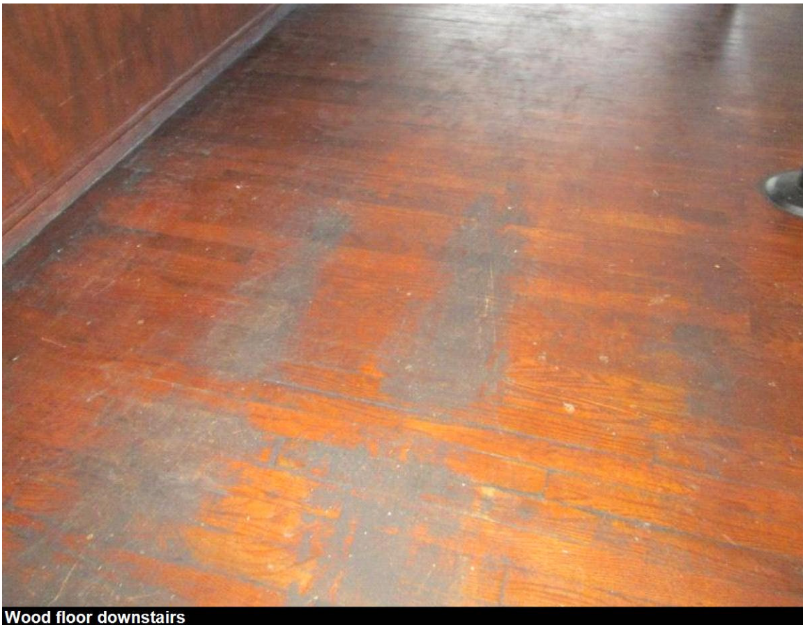
Wood floor downstairs
