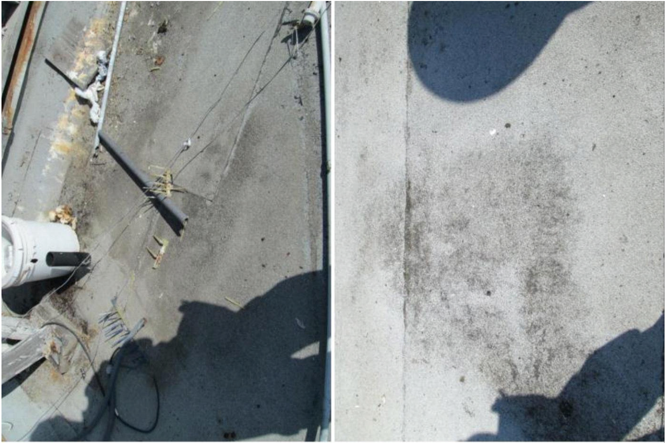
Views of roof
