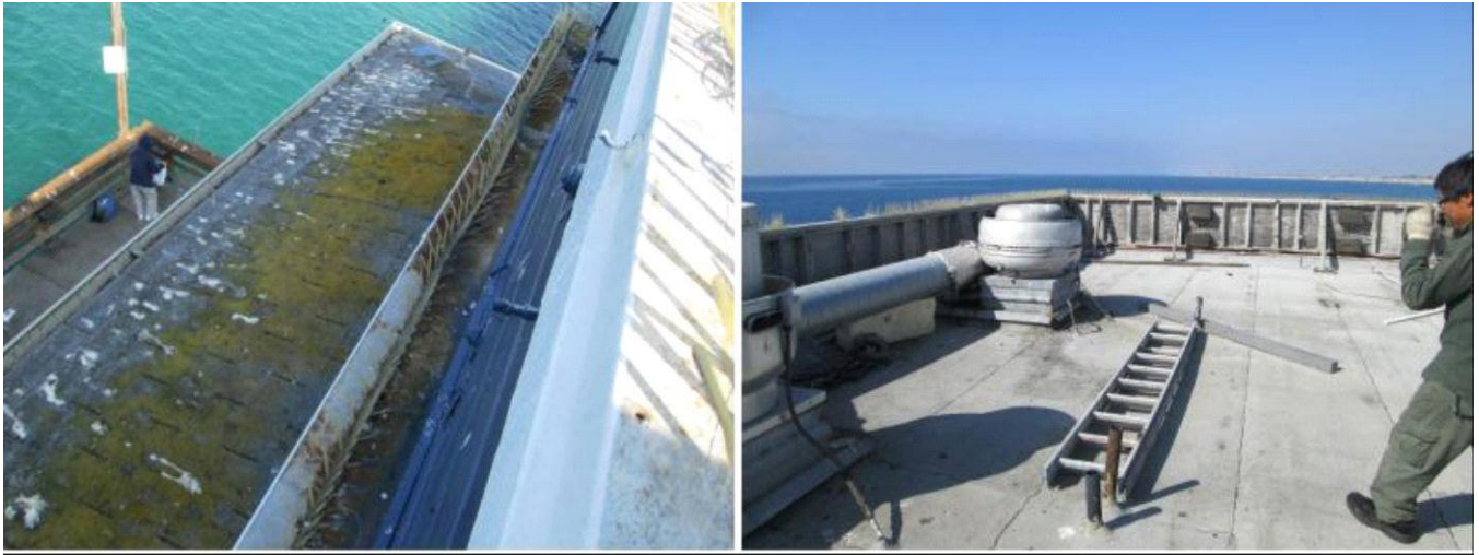
More views of roof
