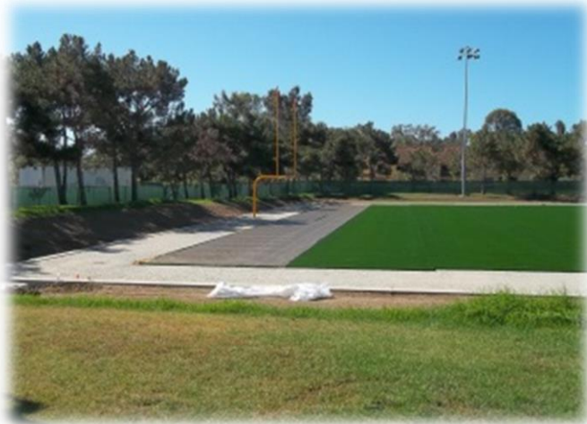
Sports field is looking good with the new turf installed.
