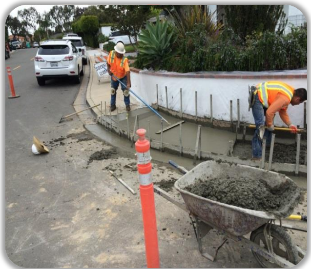
ADA Curb Access Ramp Reconstruction
