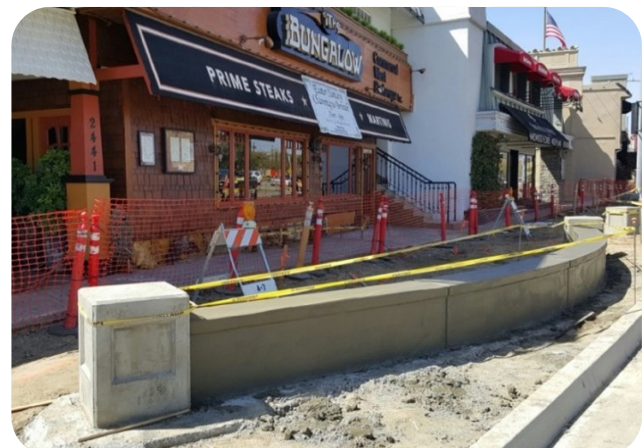
Finished Curb/Gutter, Pilasters and Seat Walls
