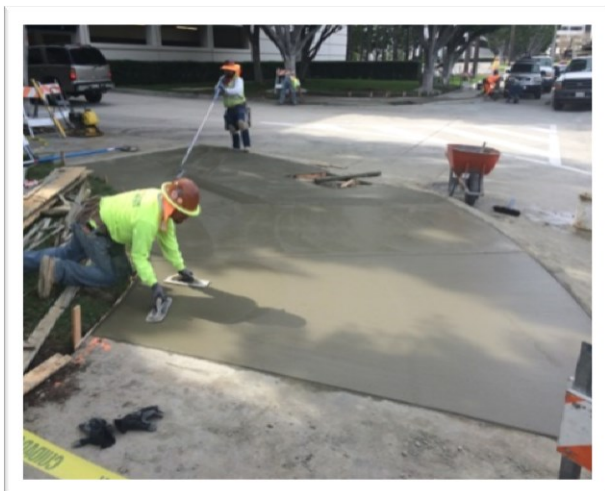
ADA Curb Access Ramp Replacement
