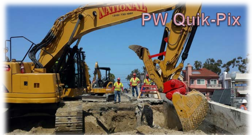
Park Avenue Bridge Demolition Photos!
