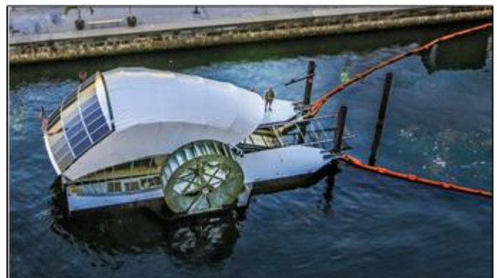
INSTALLED WATER WHEEL - BALTIMORE
