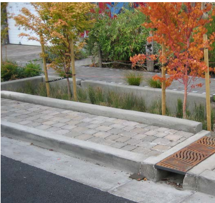
Bioswales allow stormwater runoff to infiltrate, filter pollutants out of the water, and reduce impact on traditional drainage systems
