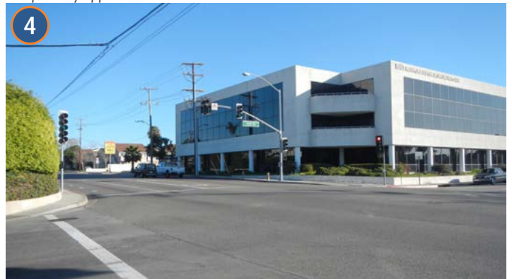
Intersection at Placentia Avenue and 15th Street looking north with crosswalk enhancement, bike lane improvements, and sidewalk improvement opportunities
