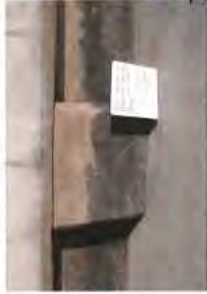
Grand Canal East, 91 ft N. of South Bay
