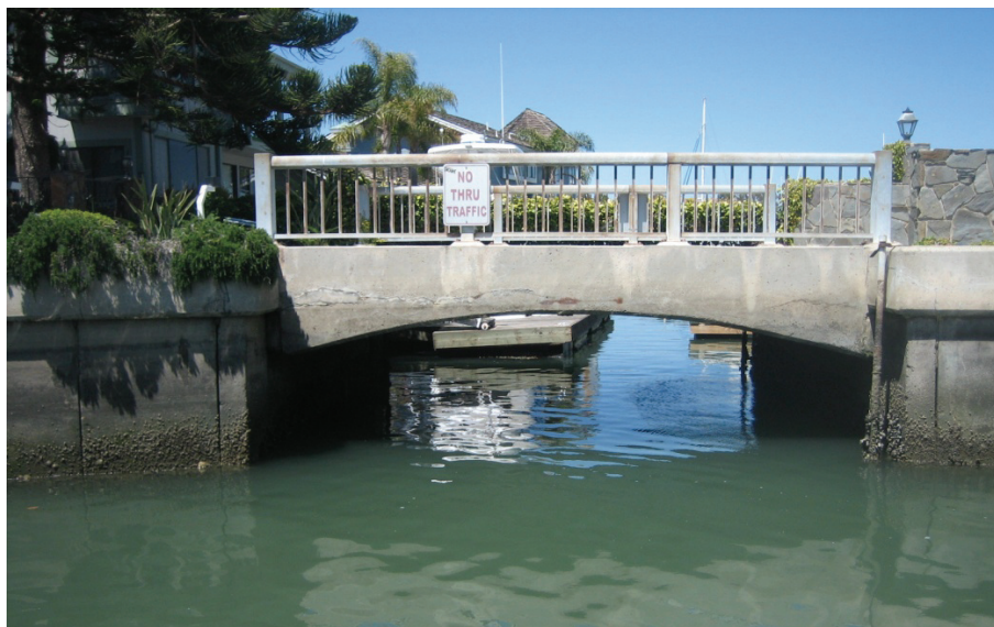
Figure 4.13 Collins Island Bridge Interface at Seawall Abutment
