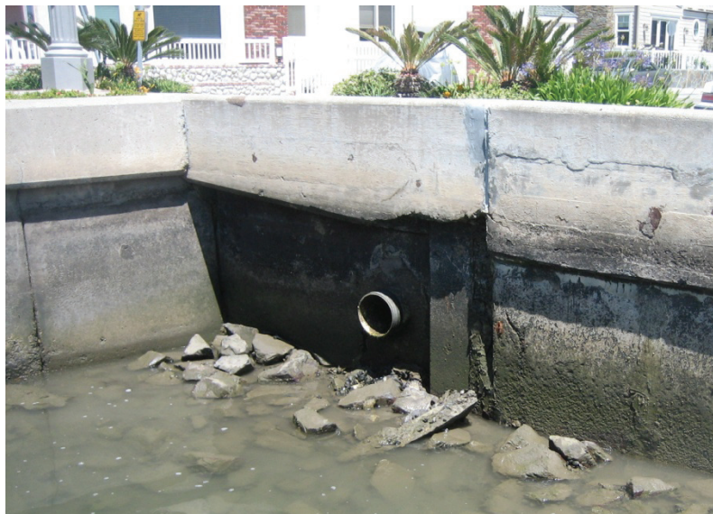
Figure 4.9 Storm Drain Outlet Through Seawall
