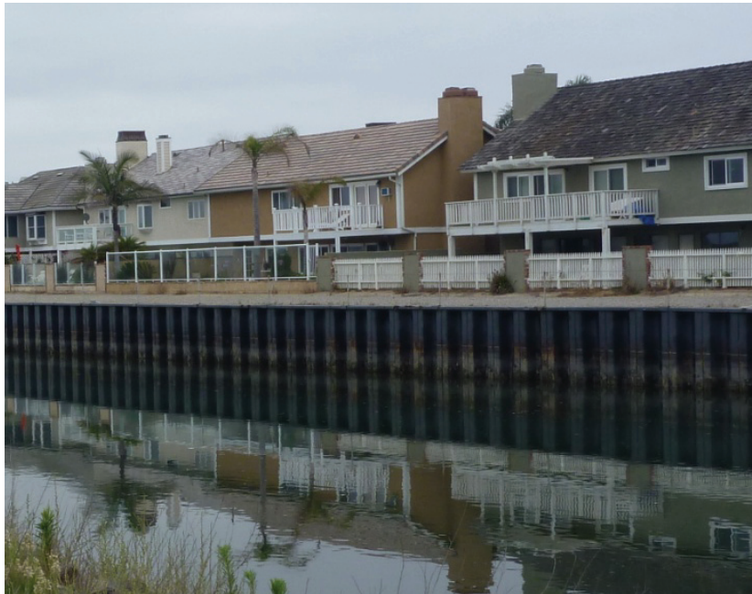
Figure 5.6 Steel Sheet Pile Bulkhead
