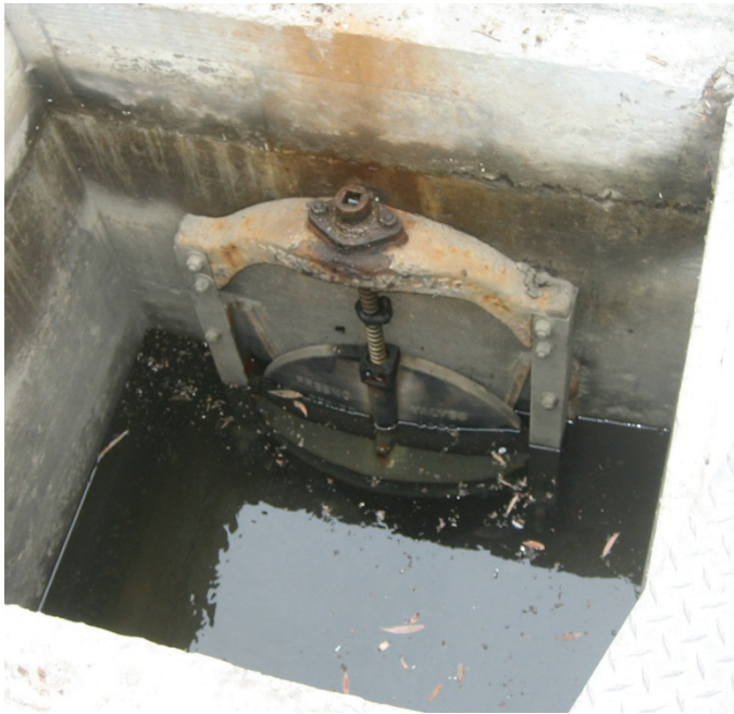
Figure 4.10 Hand-Operated Gate Valve in Storm Drain Manhole
