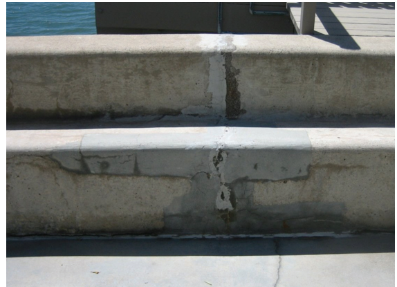
Figure 4.6 Typical Crack and Spall Repairs
