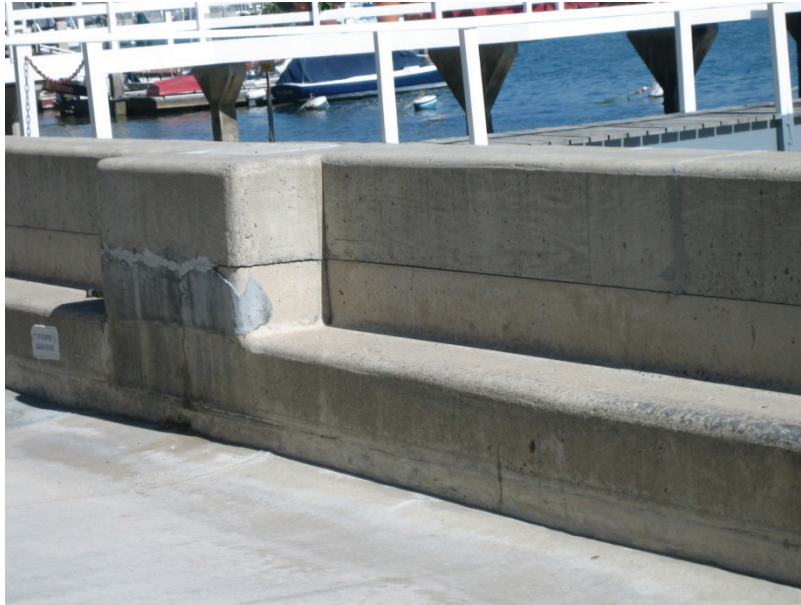
Figure 4.4 Little Balboa Seawall Cap Extension
