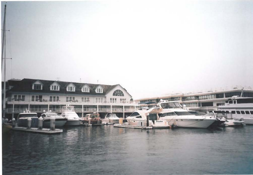
A view of a typical commercial pier along Mariner's Mile.
