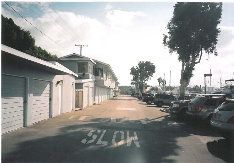
A view of the parking area at Bayside Marina. The apartments and garages are on the left with the slips and docks on the right.
