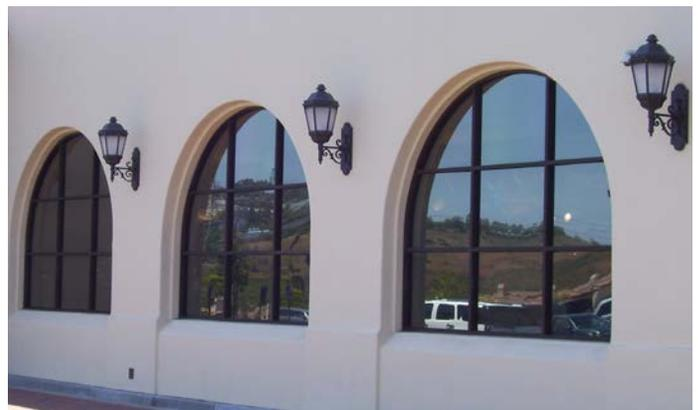
*Example of lighting with caps to prevent light from shining upward*
