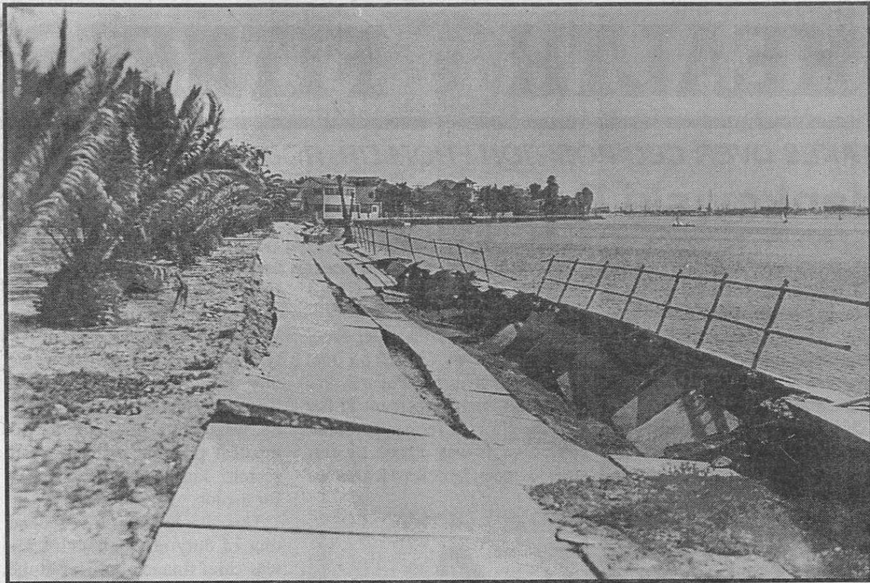
EARTHQUAKE DAMAGE. The Naples sea wall suffered extensive damage, as did much of the Long Beach area, in the 1933 earthquake. —Photo courtesy Historical Society of Long Beach
