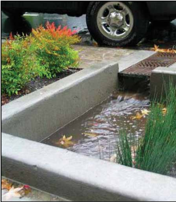
Figure 9.12 Stormwater planter, Portland, Oregon
