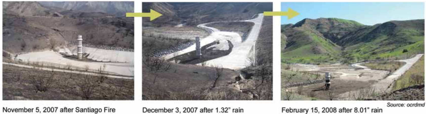
Figure 6.1 Hicks Canyon Retarding Basin sediment levels after the 2007 Santiago fire and subsequent winter rains. (3-photo sequence)
