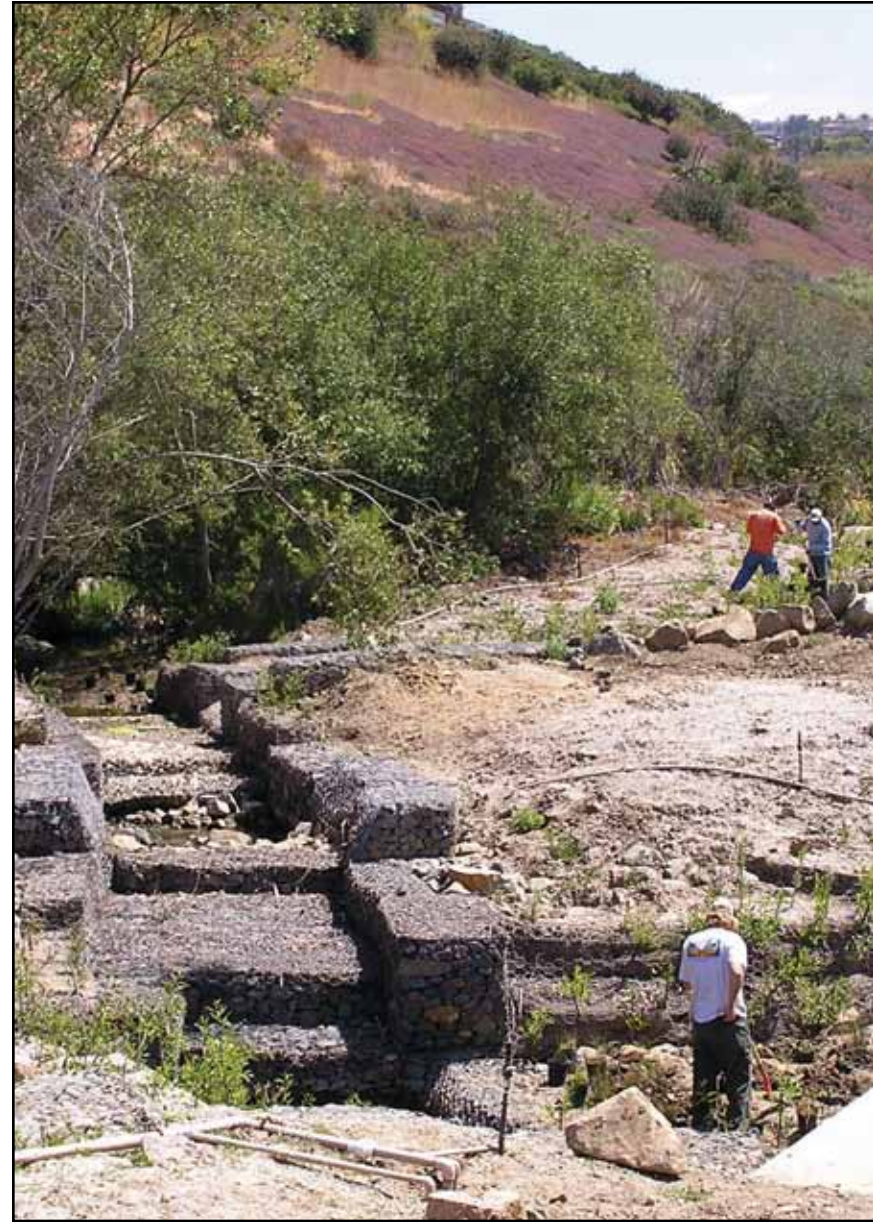
10.21 Buck Gully Road Maintenance and Wetland Project
