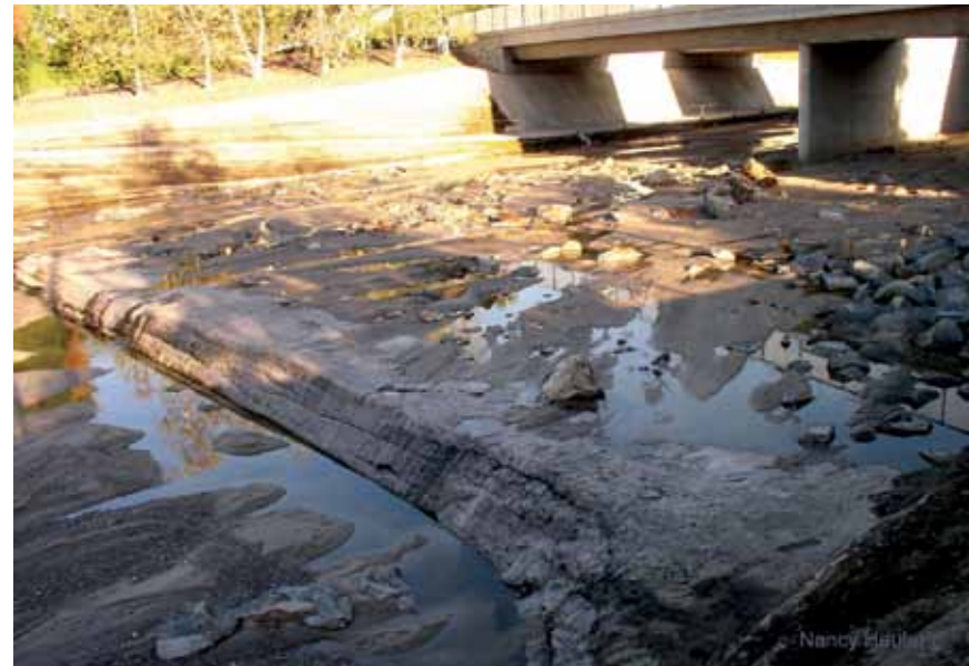
Figure 5.1 Sediment in San Diego Creek near Barranca Parkway, Irvine
