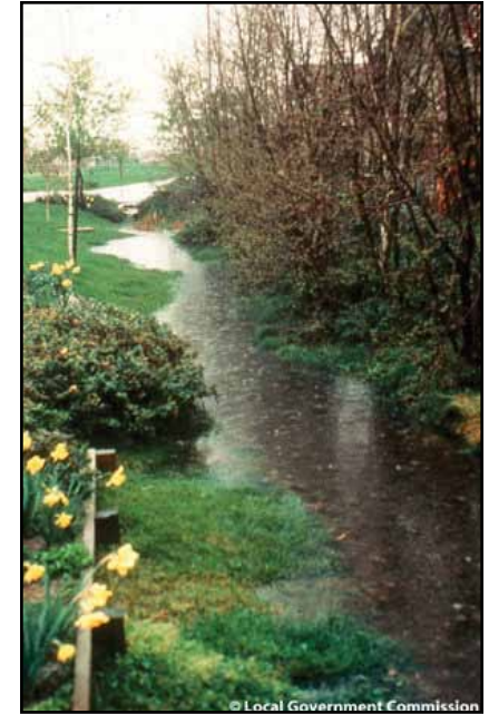
Figure 9.6. Neighborhood vegetated swale, Village Homes, Davis, California.
