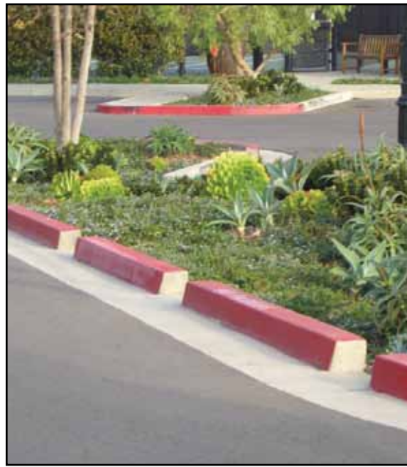
Figure 9.13 Curb cuts in parking lot median
