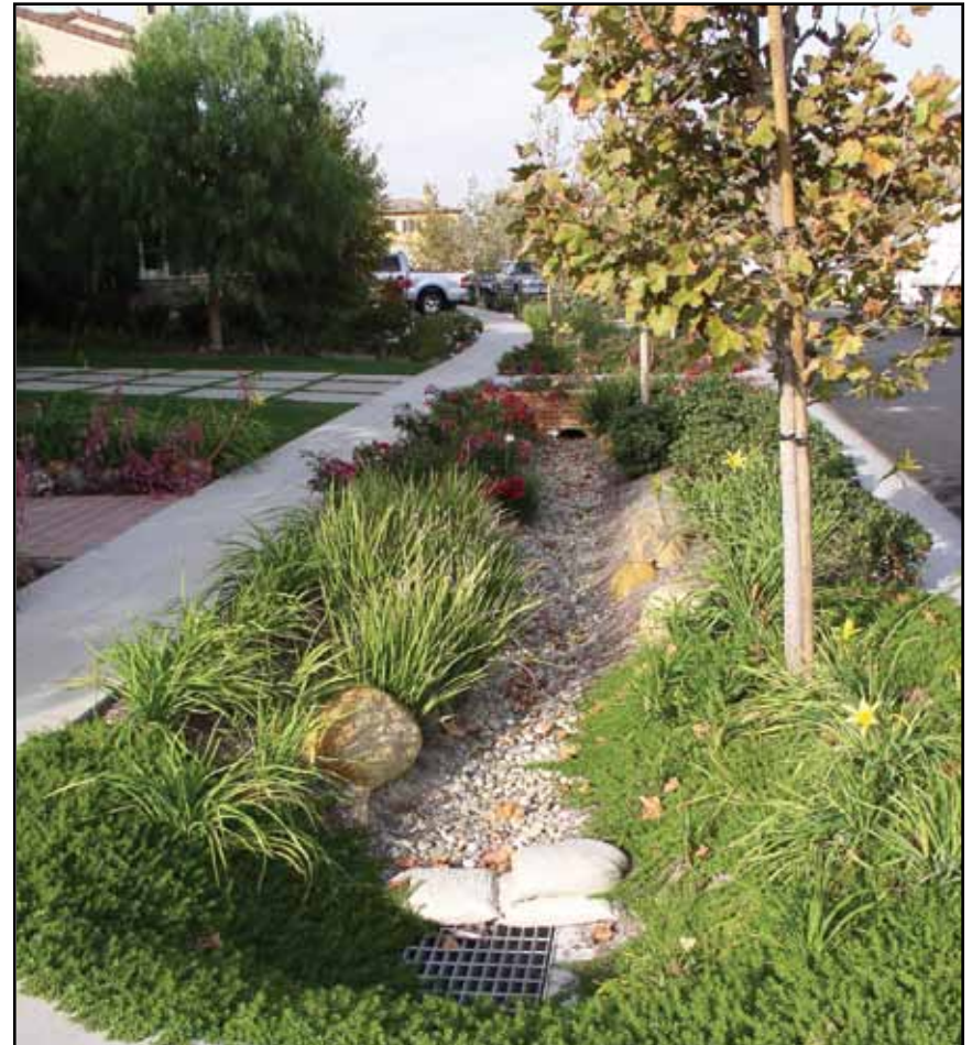
Figure 6.5 Swale at Ladera Ranch, Orange County
