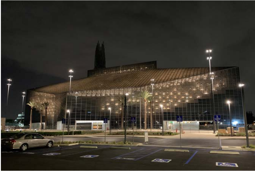
Christ Cathedral Garden Grove, CA Archdiocese of Orange County Johnson Fain Architects Rios Clementi Hale Studios
