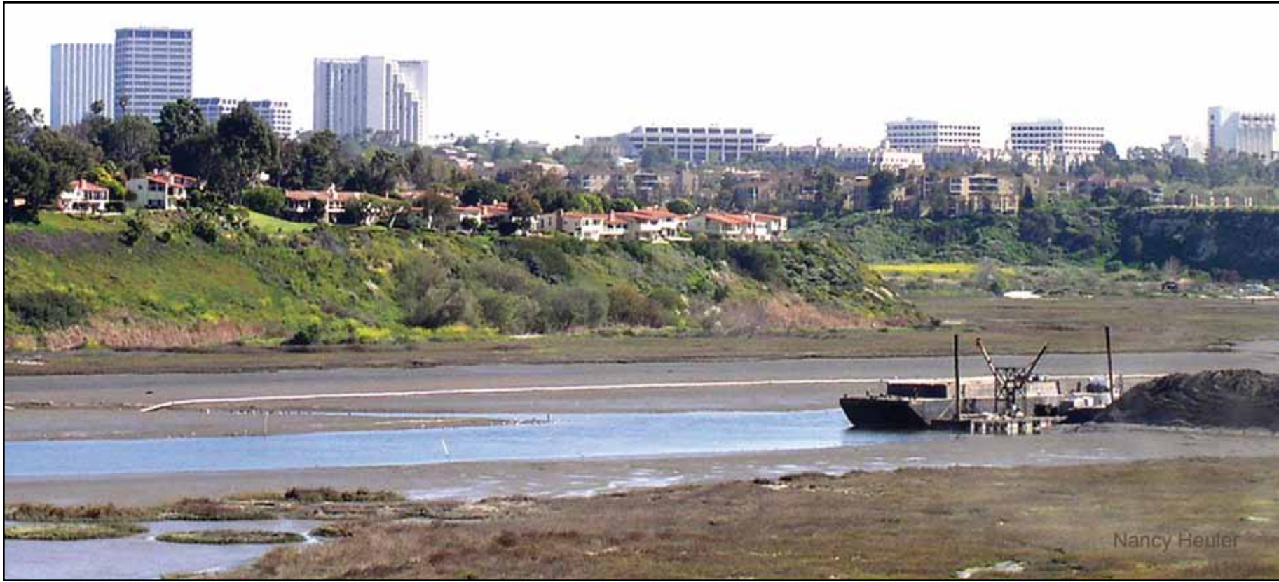
Figure 10.11 Dredging in Upper Newport Bay, Army Corps of Engineers restoration project
