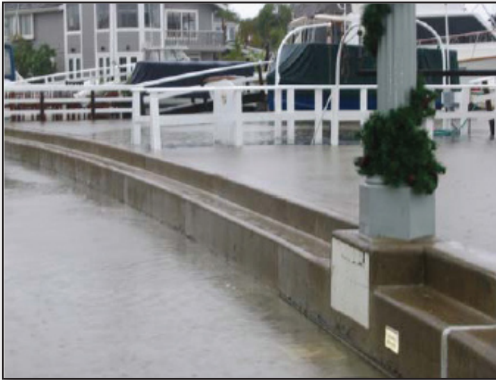
Figure 1: Photographs of the January 10, 2005 high tide that reached the 7.8 ft (MLLW) level.
