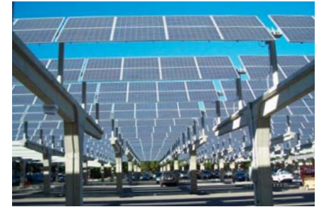
PV Arrays as Parking Lot Shading
