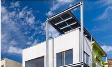
Integrated solar panels
