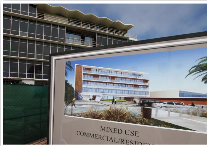
Renovations Under Way Within lido Village
