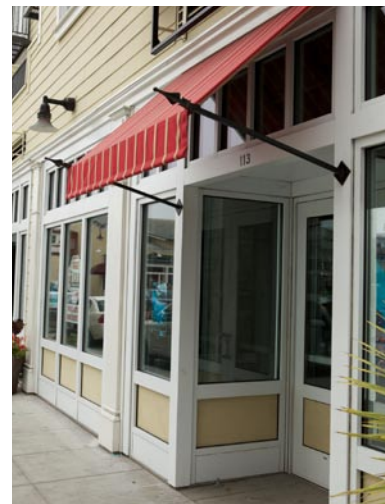
Natural material emphasis at ground
