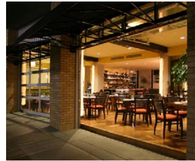
Retractable doors on restaurant
