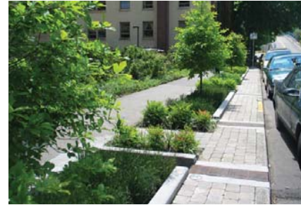
'Green Street' Bioswale
