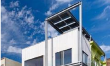
Integrated Solar Panels
