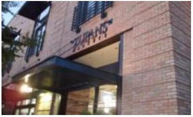
Metal Awning Shelters Entrance
