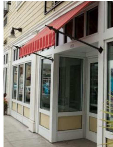
Natural Material Emphasis at Ground
