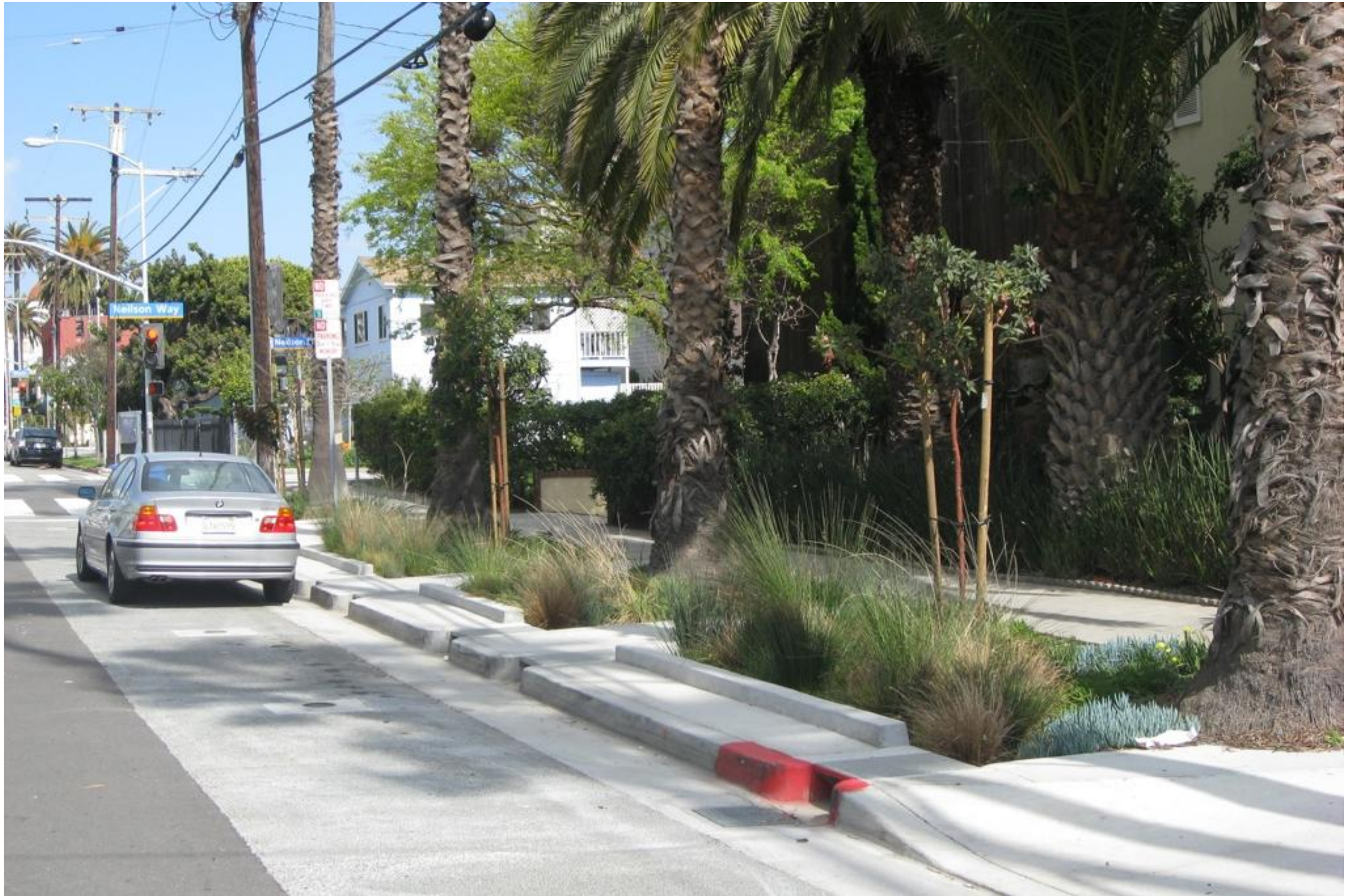
Porous Concrete on Street in Parking Zone
