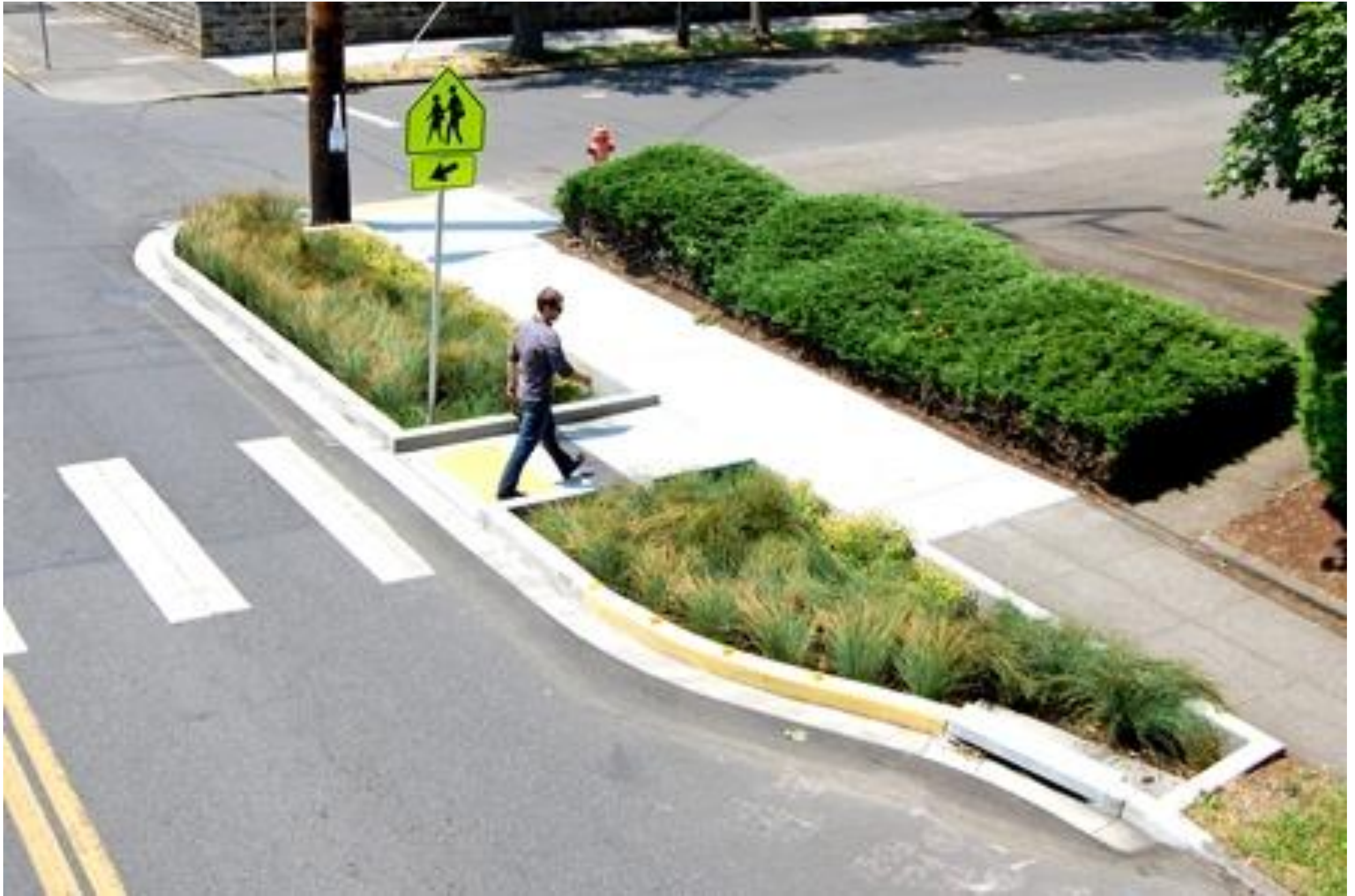
Residential Landscaped Curb Extension
