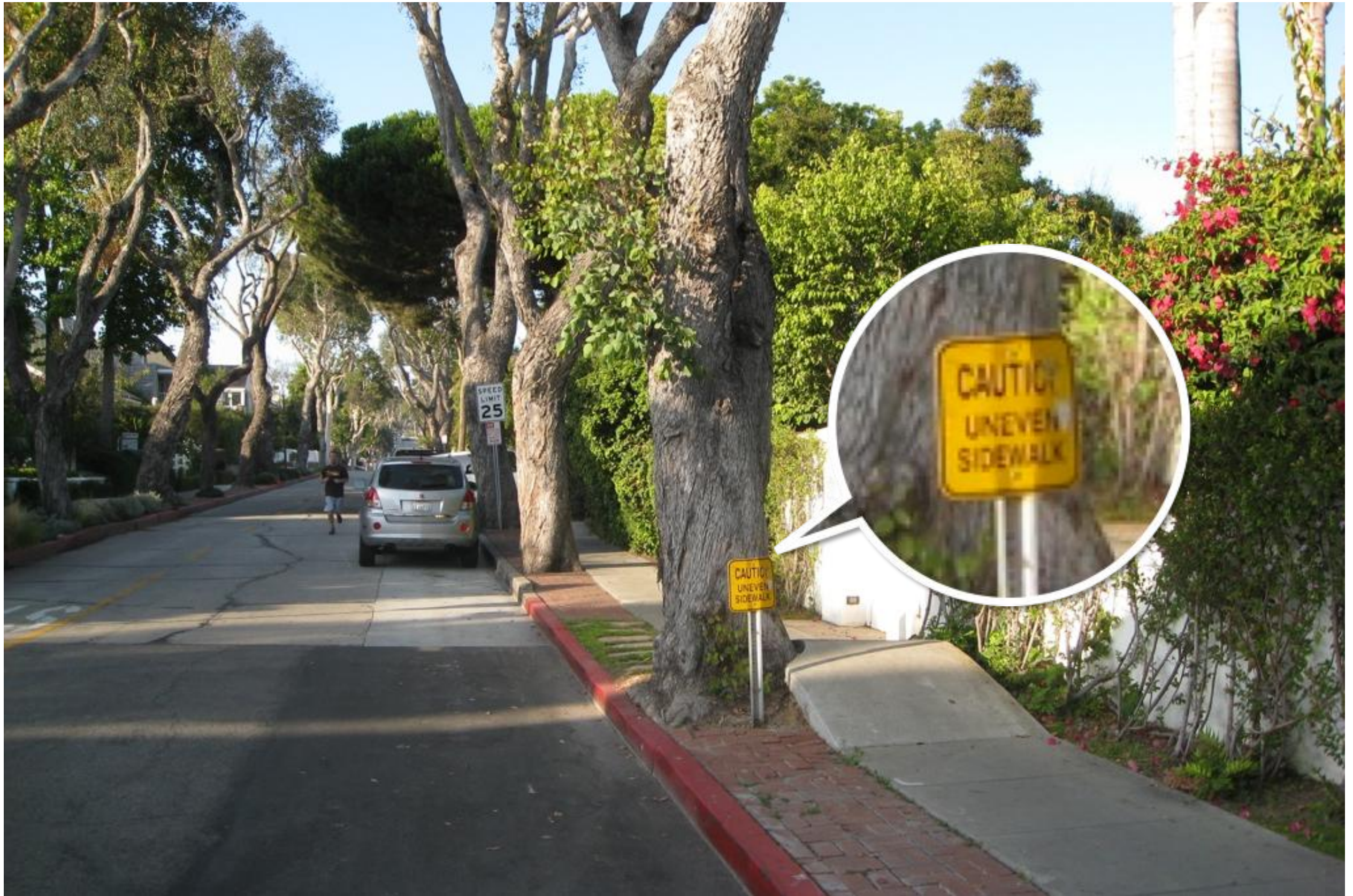
CAUTION: Uneven Sidewalk
