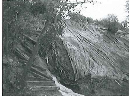
1997 Slope Failure in Morning Canyon
