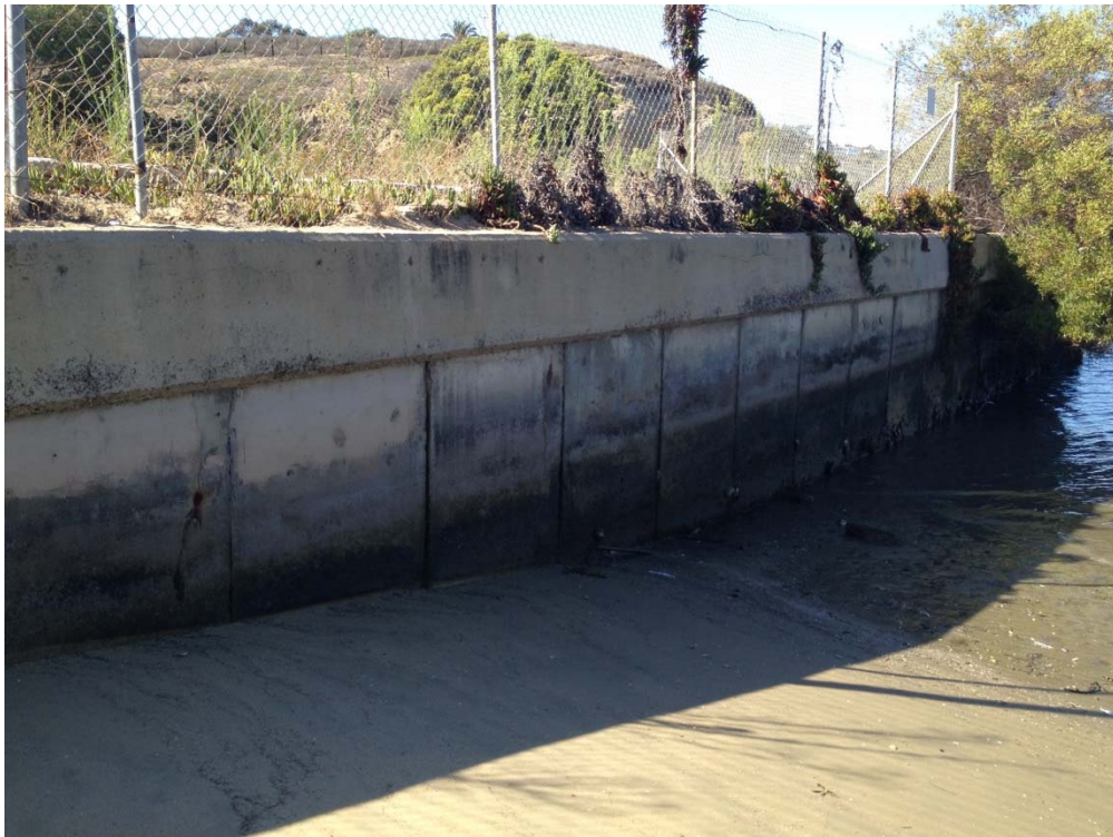
Photograph 4. Southern stretch of wall.
