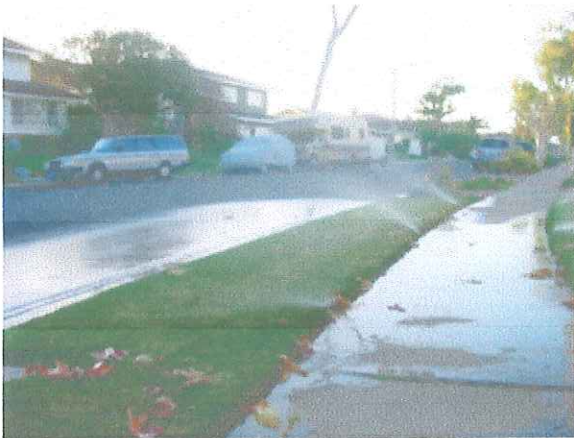
Figure 2. Sprinklers overshooting lawn onto street
