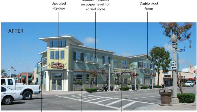
Removed existing mansard roof and add second story Added stone bulkheads
