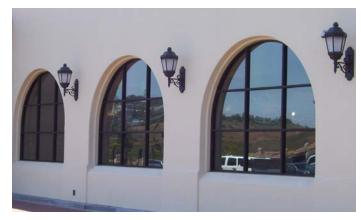
Example of lighting with caps to prevent light from shining upward
