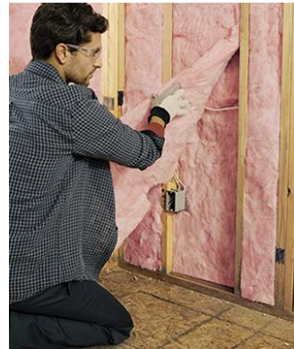
Quality Insulation Installation
