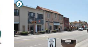
BALBOA BOULEVARD EXISTING CONDITIONS
