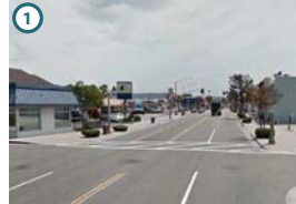
BALBOA BOULEVARD EXISTING CONDITION
