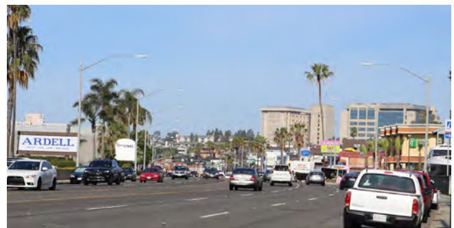
Dangerous Ped Crossing
