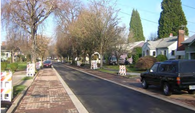
Permeable Pavers in the Parking Lane
