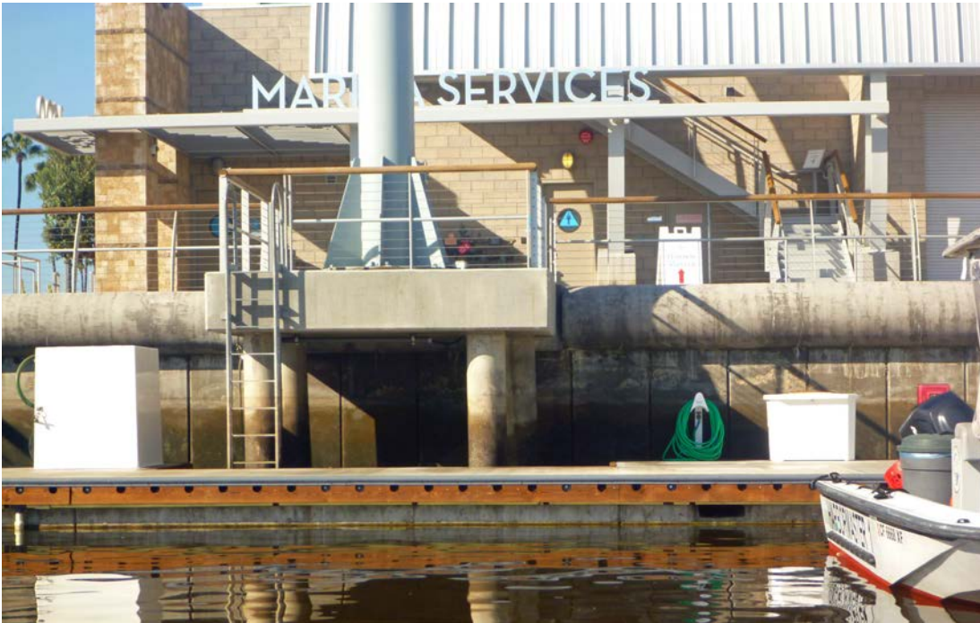
Figure 7 New City Seawall – Example of Level 1 Condition
