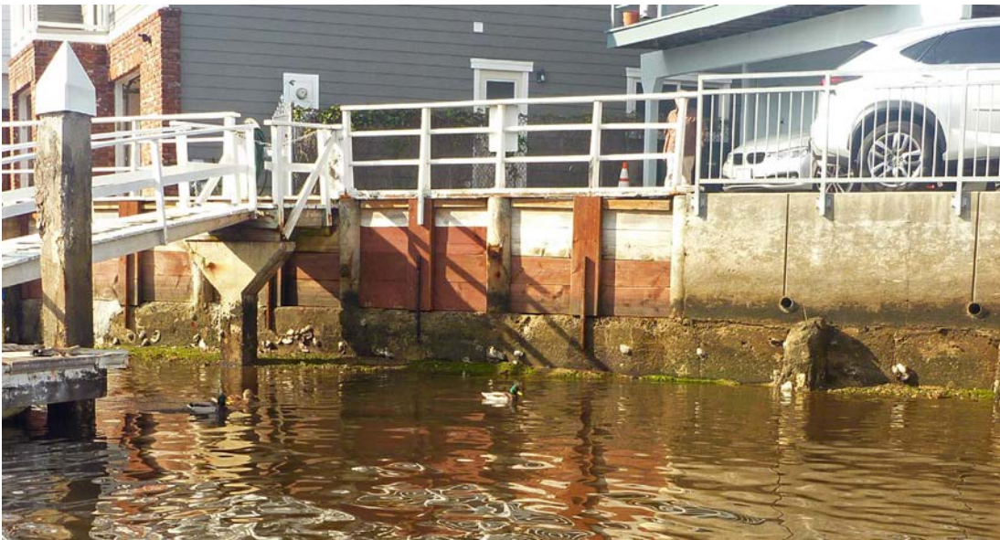
Figure 12 Residential Seawall – Level 3 Condition
