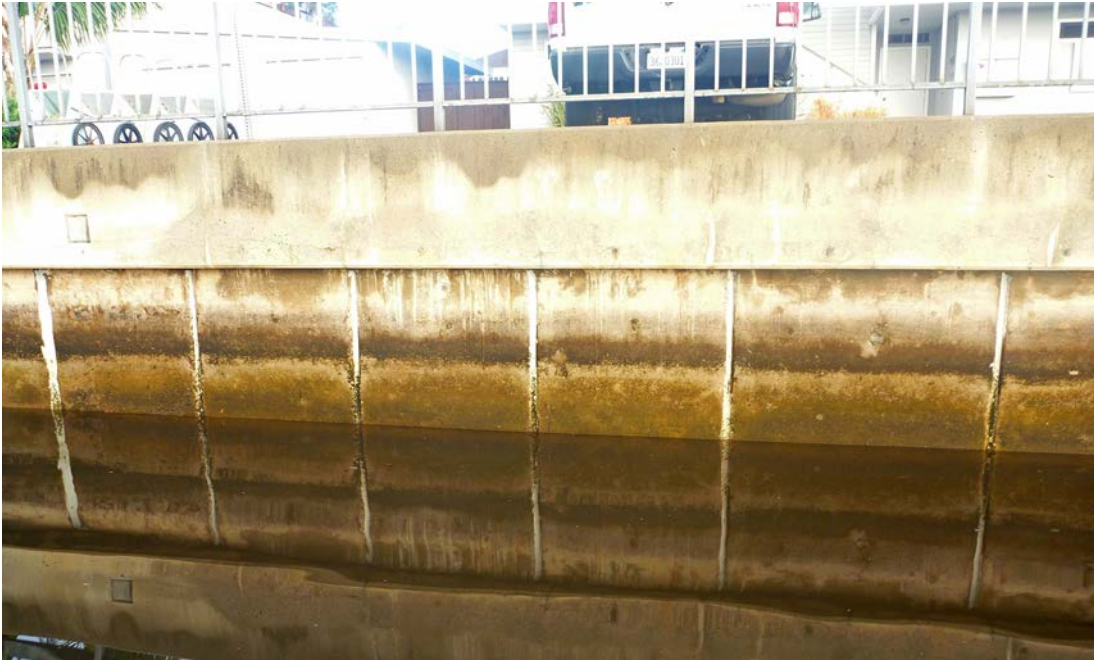
Figure 6 Well-Maintained City Seawall – Example of Level 1 Condition
