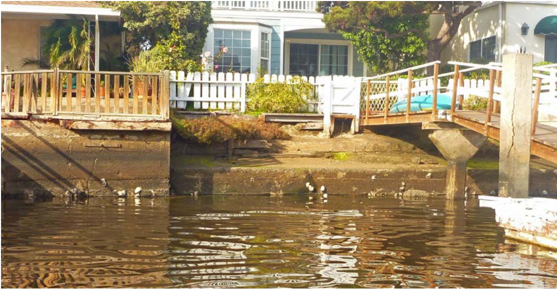
Figure 11 Residential Seawall – Level 3 Condition
