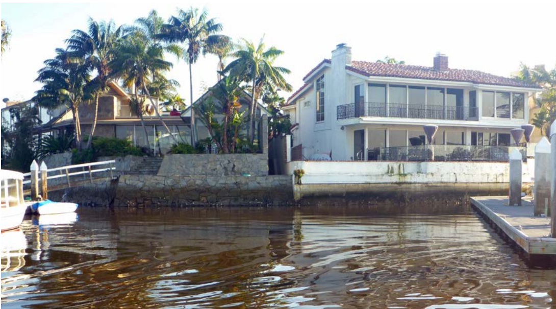
Figure 10 Residential Seawall Cap Extension – Level 2 Condition
