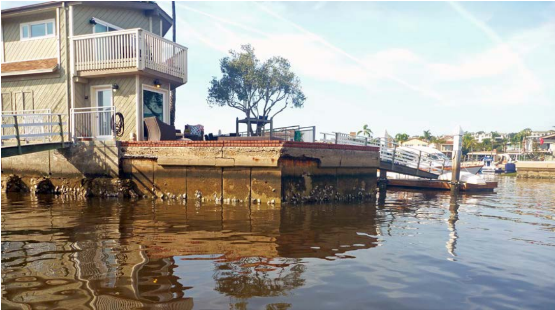
Figure 9 Residential Seawall Cap and Extension – Level 2 Condition
