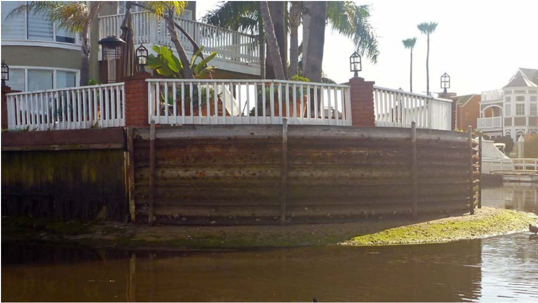
Figure 13 Residential Seawall – Level 3 Condition
