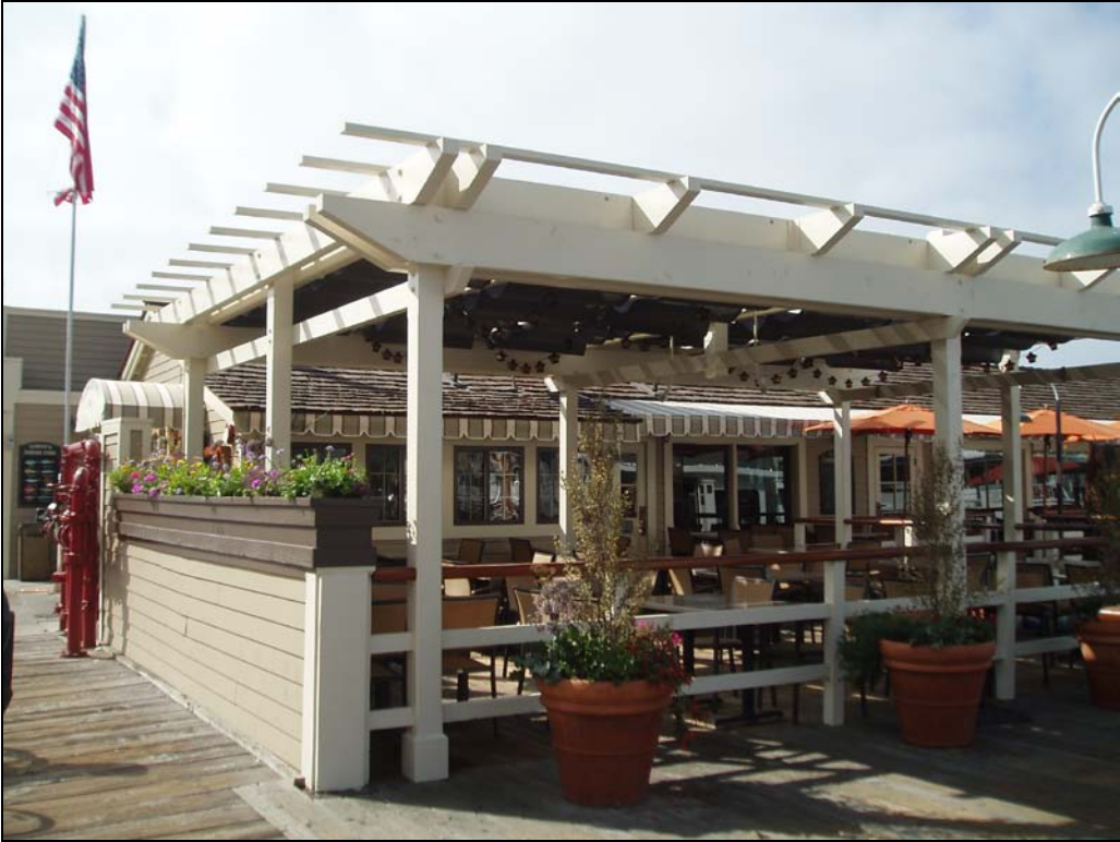
Bluewater Grill, Patio Structure
