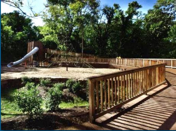
Accessible Wood Ramp
