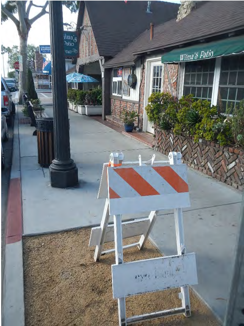
Empty tree well between 201 and 207.
