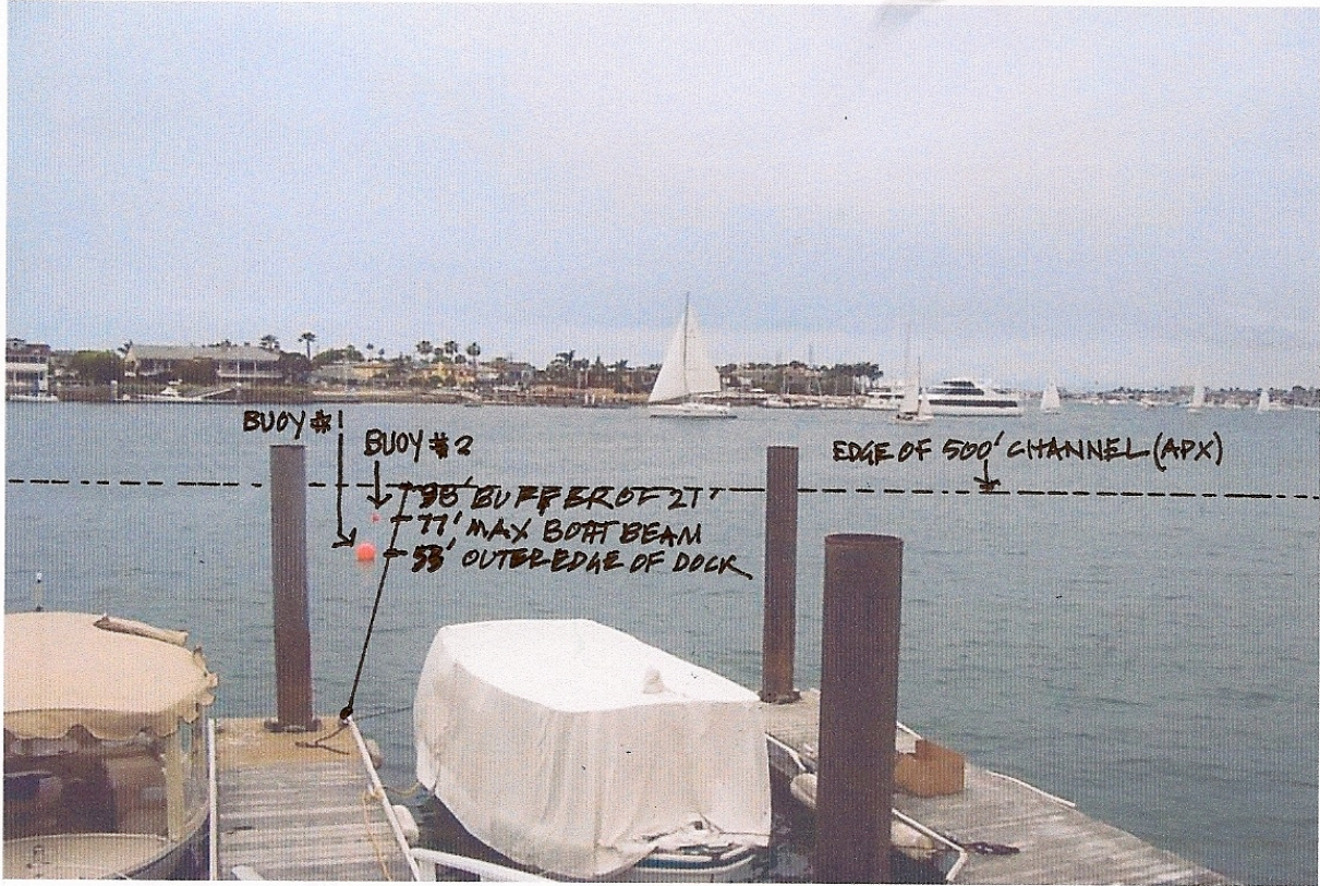
Buoys #1 & # 2 and Existing Docks , View From Pier End
