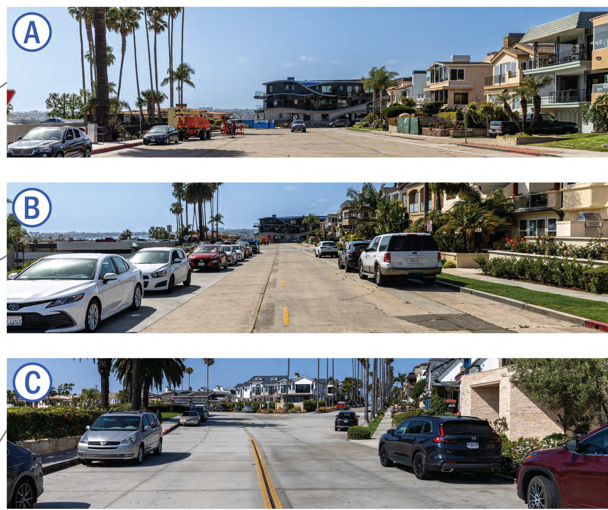
A Street Cross Section has been provided for the pictures which contain a letter reference. Refer to sections on the right.
