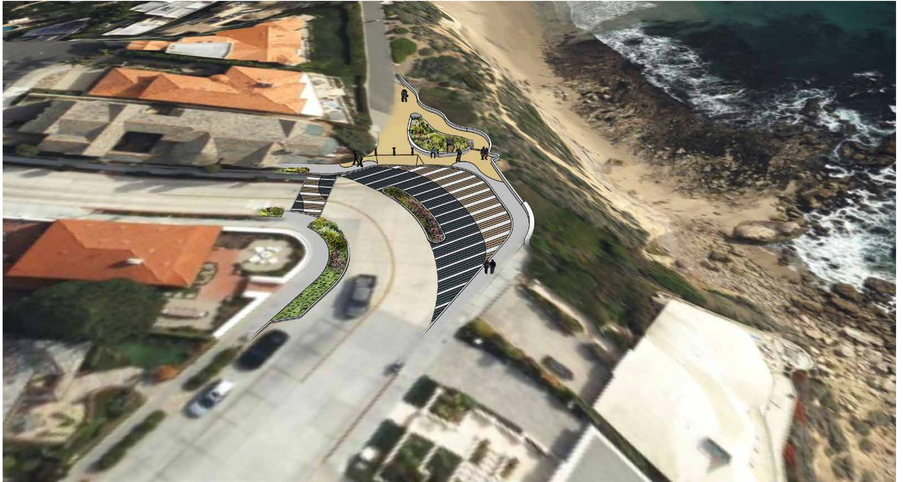
Aerial view overlooking Little Corona drop-off looking south along the coast.
