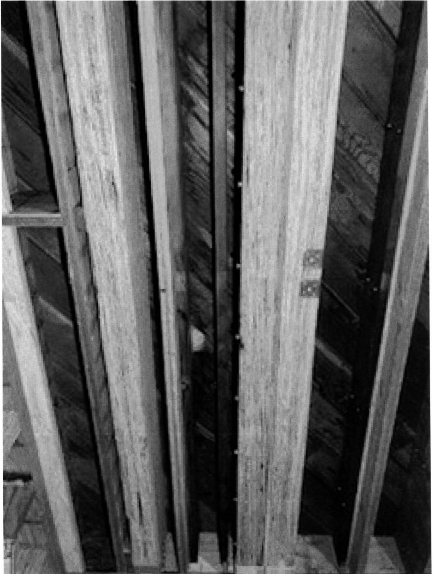
First floor ceiling – Interface between new and legacy joists
