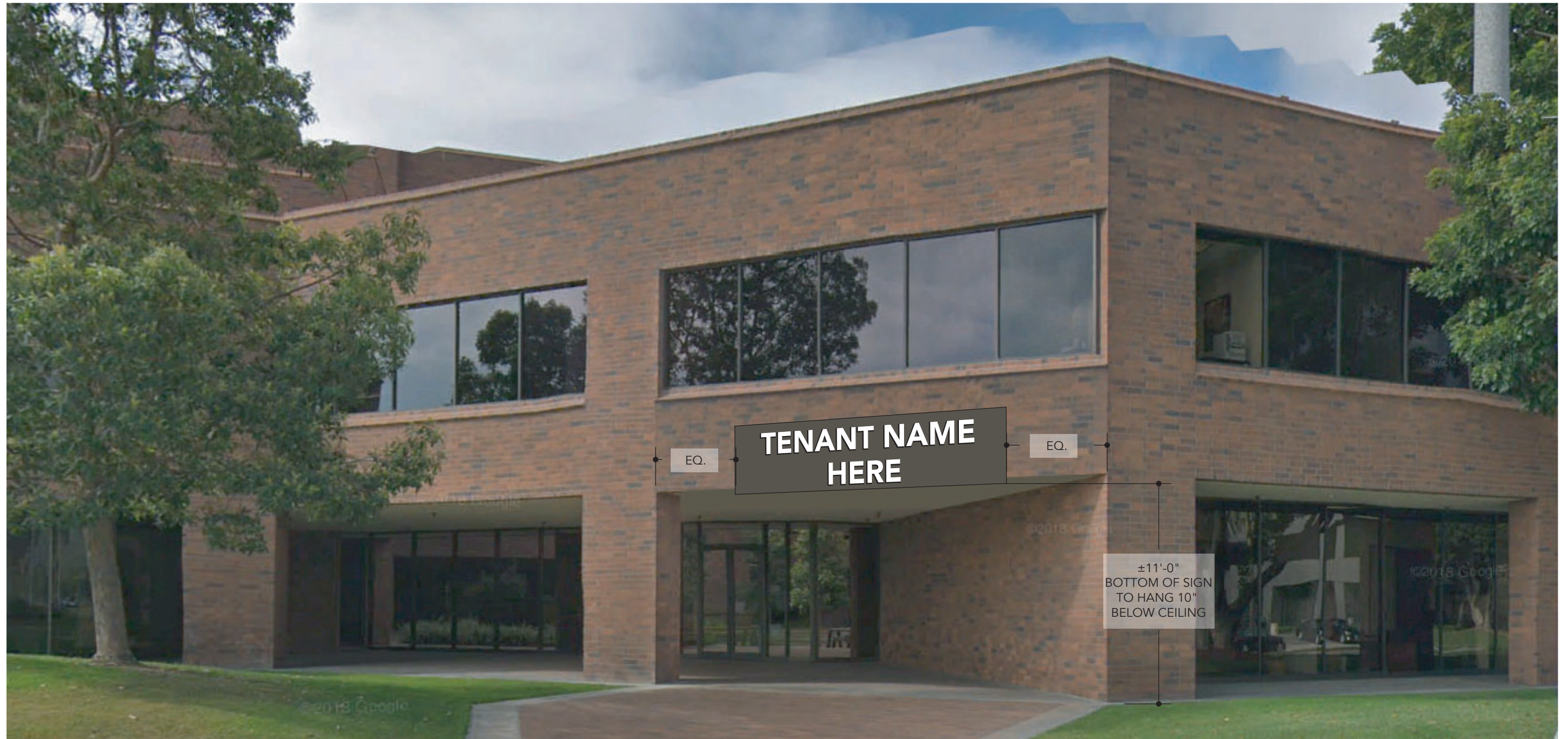
NORTHEAST ELEVATION VIEW - 4041 MACARTHUR BLVD. (SIGN NO. 3.2)
