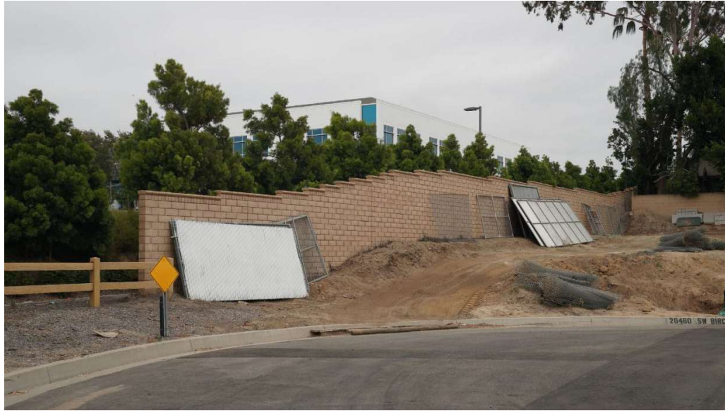
IMAGE 6 RETAINING WALL AT ADJACENT LOT
