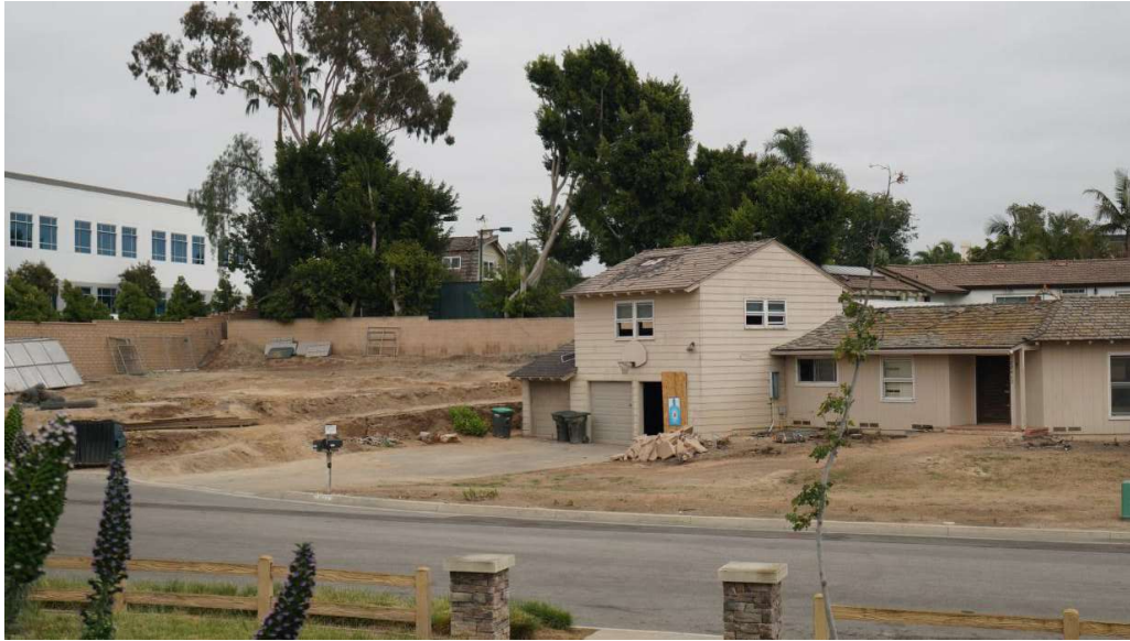
IMAGE 1 GARAGE ON SUBJECT PROPERTY GRADED SUBSTANTIALLY LOWER THAN ADJACENT LOT
