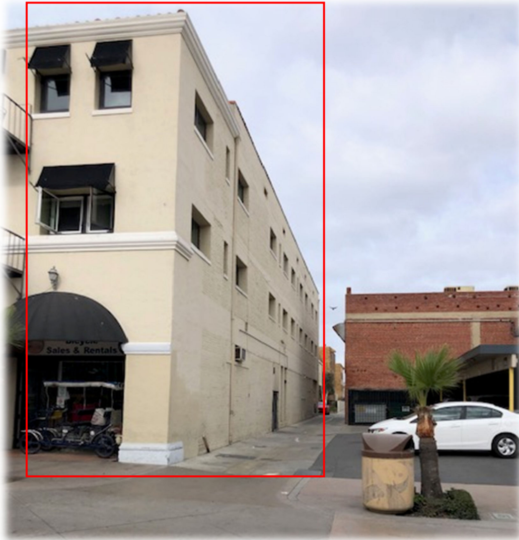
Side of rear area, showing the bed and breakfast building at the rear of BT
