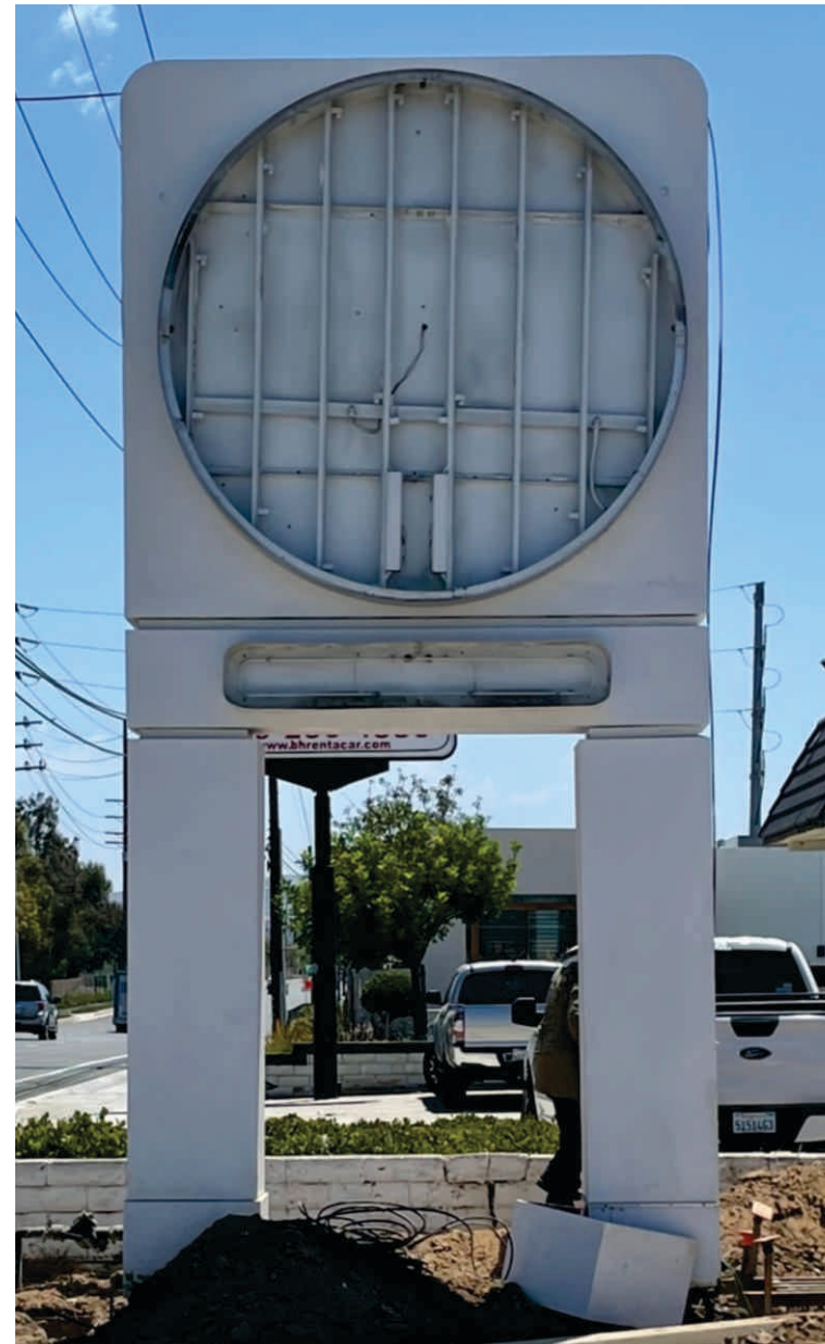
EXISTING PYLON SIGN CONDITIONS
